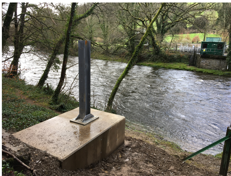
Figure 3: Image showing the presence of a new cableway stanchion installed in February 2020 (after the end of the field experiment documented here).
