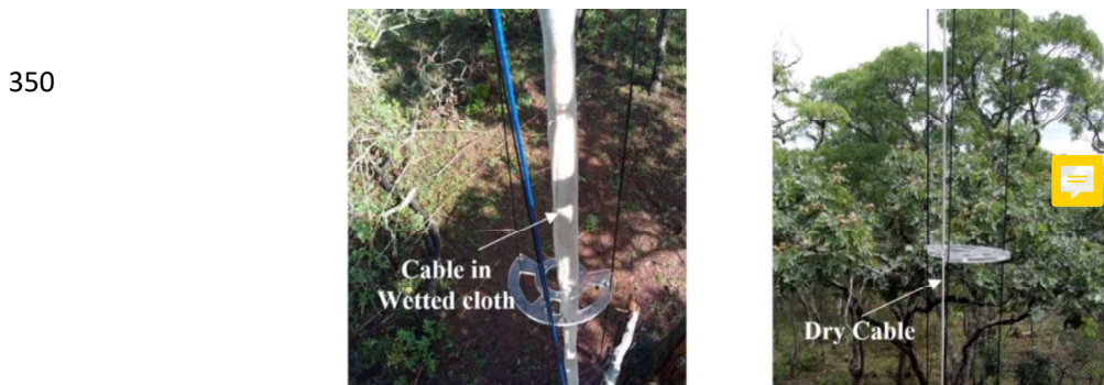
Figure 3. Installing the wet (left) and dry (right) fibre optic cable on the observation tower at Mpika site, Zambia. Under canopy view without screens.
