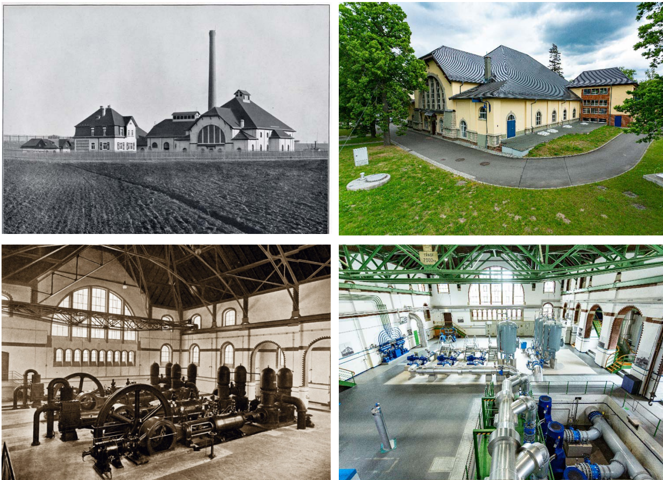
878 Figure 14: Buildings and pumps of the Canitz water works then and now, Leipzig: (left) as planned and designed by Adolf and 879 Günther Thiem, status 1912, (right): status today (Photos: Leipziger Gruppe, with permission).
