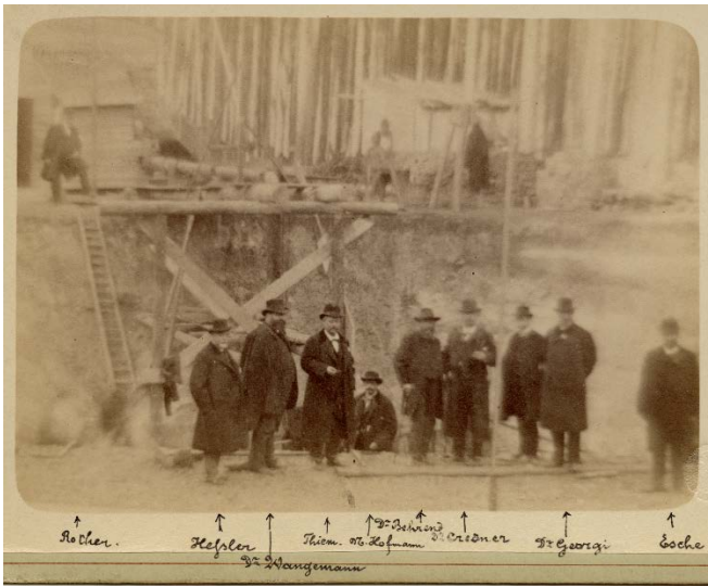
328 Figure 4: Construction of a “Ringbrunnen” at Leipzig-Naunhof, around 1887. Upper left: drilling of vertical wells, upper right: view 329 of the radial pipelines connecting the vertical wells (visible at the end) to the central collector shaft, lower left: Adolf Thiem visiting 330 the construction site (third from left, lower row). Also present is Prof. Credner, head of the Saxonian Geological Survey and Max 331 Rother (left), one of Thiem’s pupils (Photos: Stadtarchiv Leipzig).
