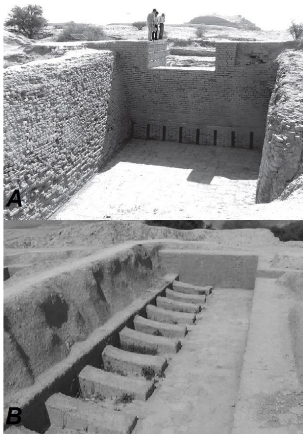
Figure 3. The remaining of the water treatment system in “Chogha Zanbil” Complex, Khuzestan, Iran; (A) Front Side View, (B) Back Side View (Adopted from Naghsh Avaran Toos Consulting Engineers Company, 2013).
