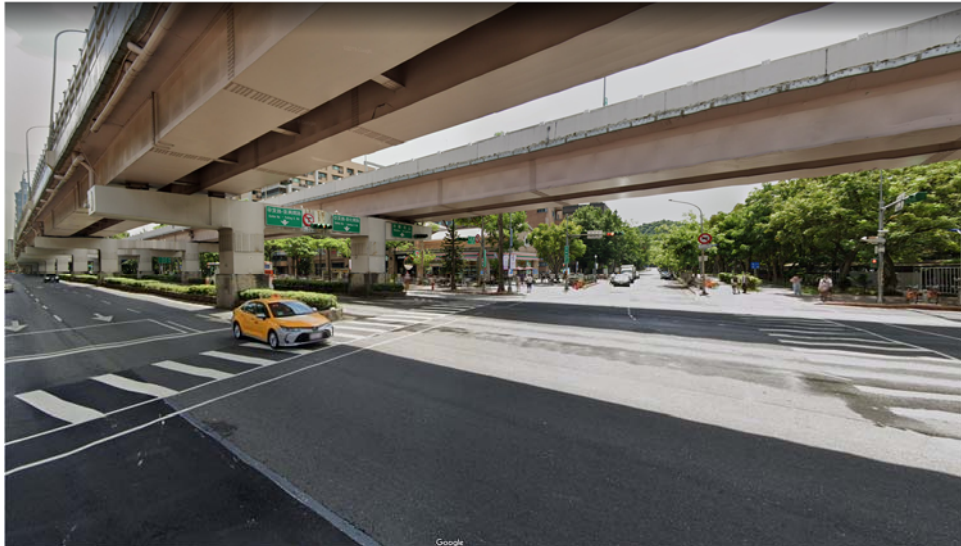
Fig. 1 The freeway is elevated and supported by the pillars at the centerline of the Keelung Road
