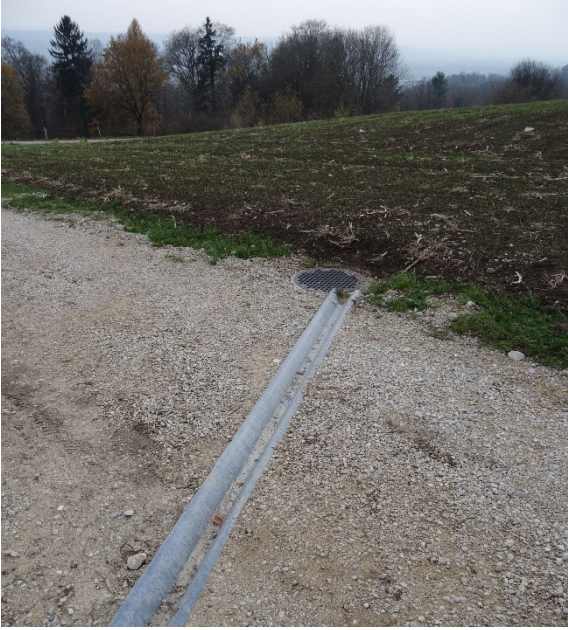
1125 Figure S 12: Channel drain and inlet with a metal grid lid on a road in the study area Lommiswil
