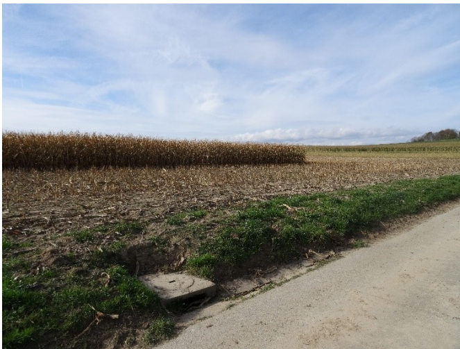
1091 Figure S 3: Lateral concrete storm drainage inlet next to a road in the study area Molondin
