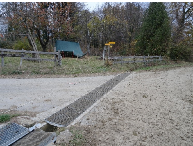
1122 Figure S 11: Channel drain on a road in the study area Clarmont
