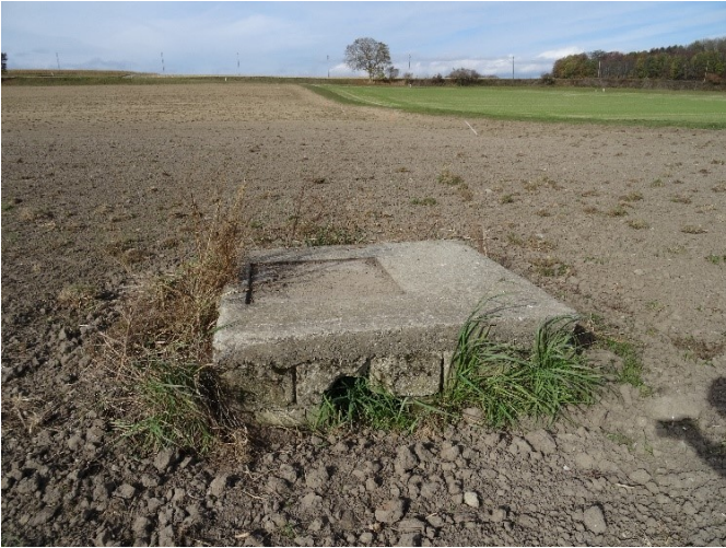
1118 Figure S 10: Tile drainage maintenance manhole in a field in the study area Molondin
