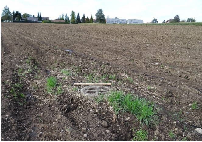
1098 Figure S 6: Storm drainage inlet with a concrete grid lid in a field of the study area Nürendorf
