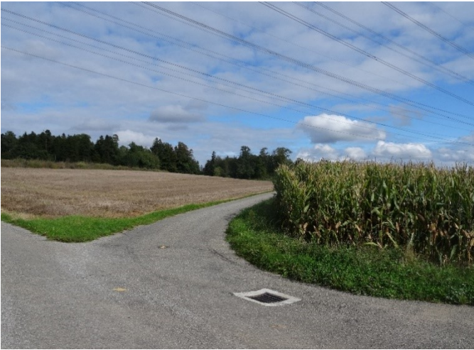
1085 Figure S 2: Storm drainage inlet with a gridded metal lid on a road in the study area Nürens Dorf
