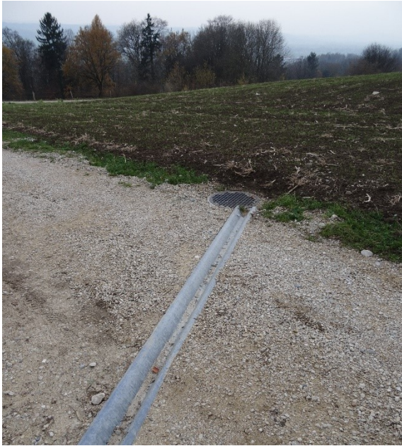
1122 Figure S 12: Channel drain and inlet with a metal grid lid on a road in the study area Lommiswil
