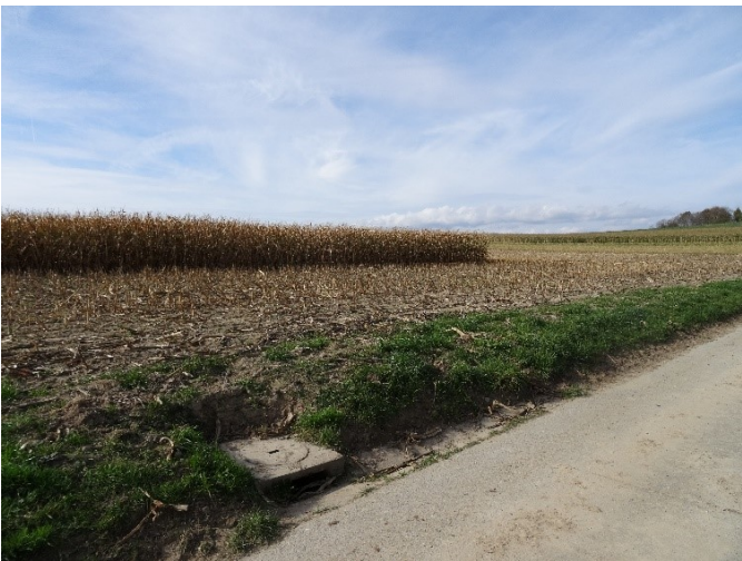
1088 Figure S 3: Lateral concrete storm drainage inlet next to a road in the study area Molondin
