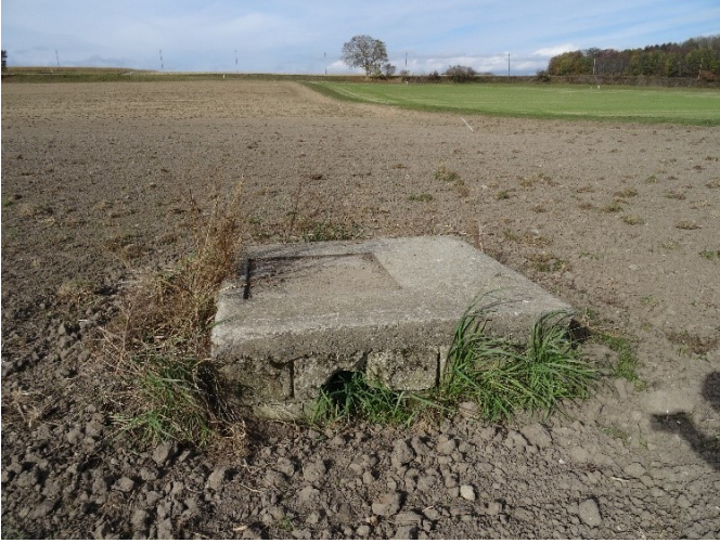
1115 Figure S 10: Tile drainage maintenance manhole in a field in the study area Molondin
