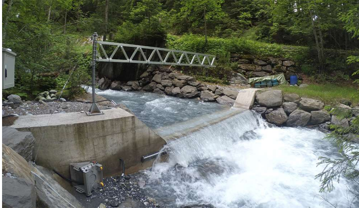
Figure-. River stage measure at the outlet. The streamflow is here measured between 0.96 and 1.13 \text{ m}^3 \cdot \text{s}^{-1} .
