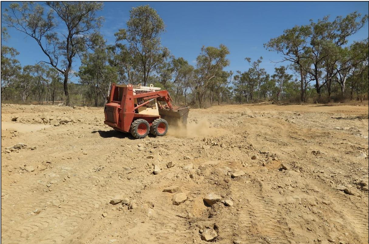
Figure S1-F. Rock capping remediated gully.
