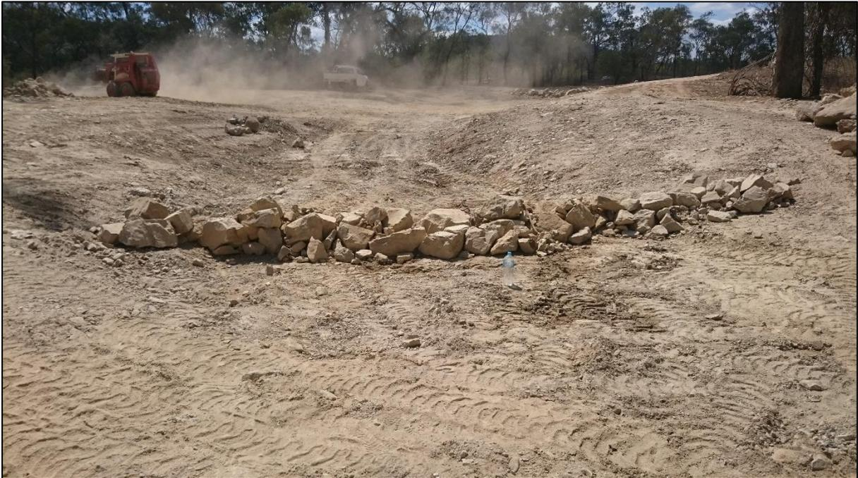
Figure SI-1G. Remediated gully completed with check dams 2016.
