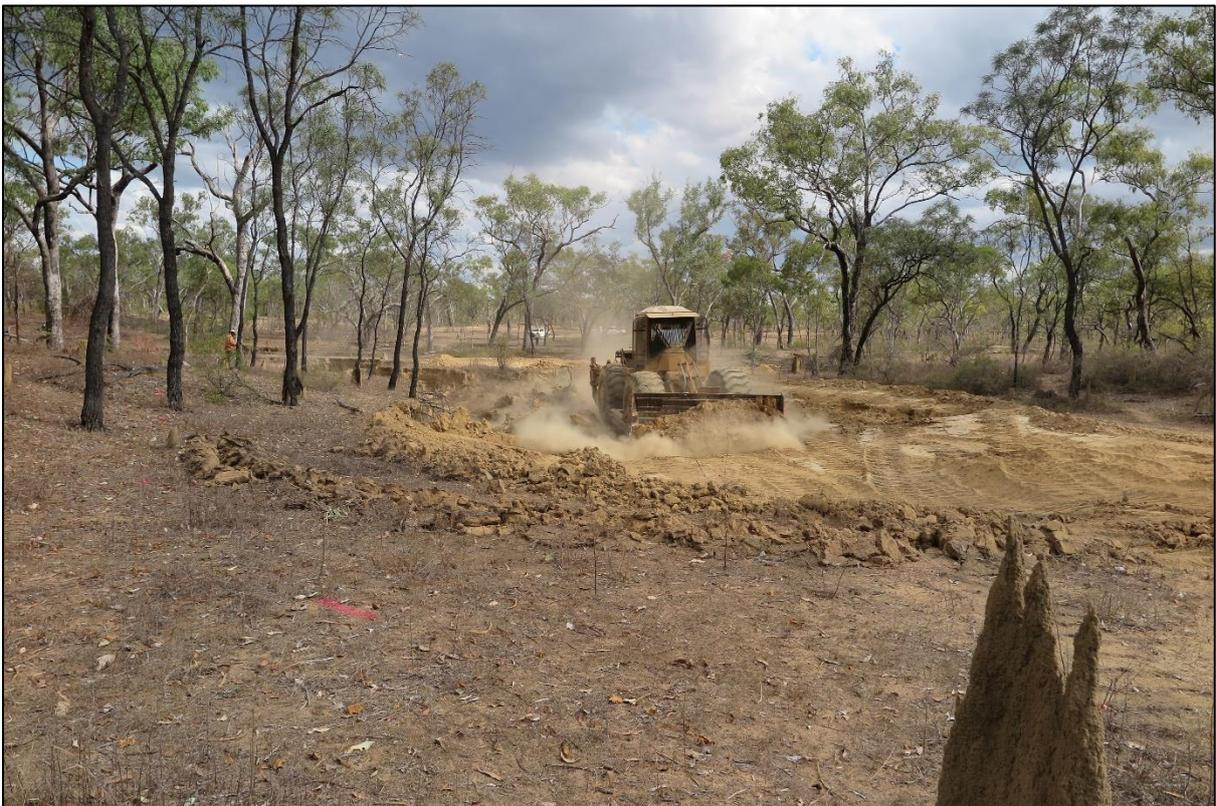
Figure SI-1B. Reshaping the remediated gully.
