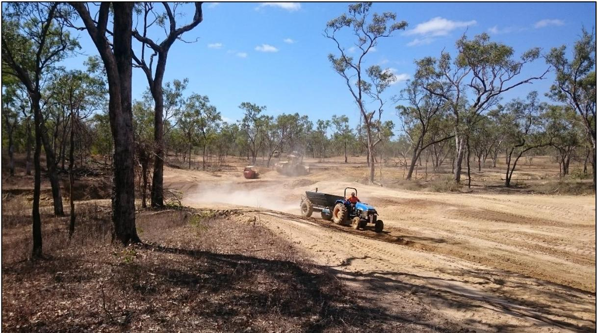
Figure S1-D. Spreading gypsum over remediated gully.
