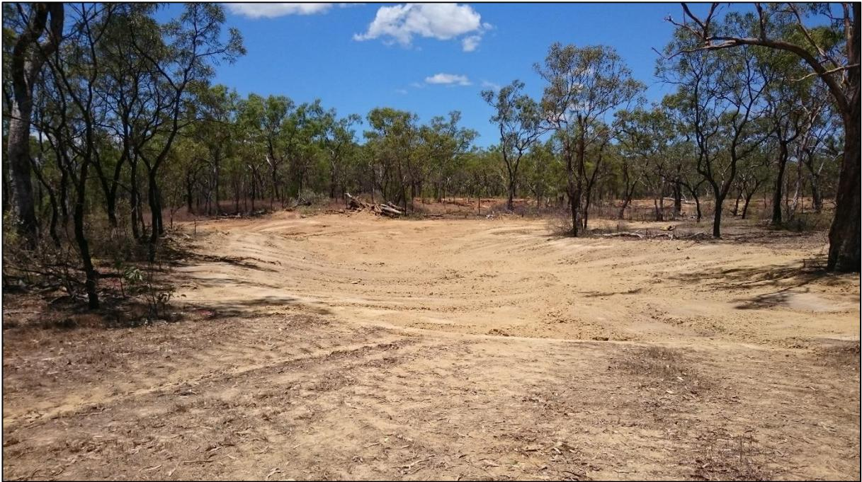
Figure S1-C. Finished reshaping of remediated gully.
