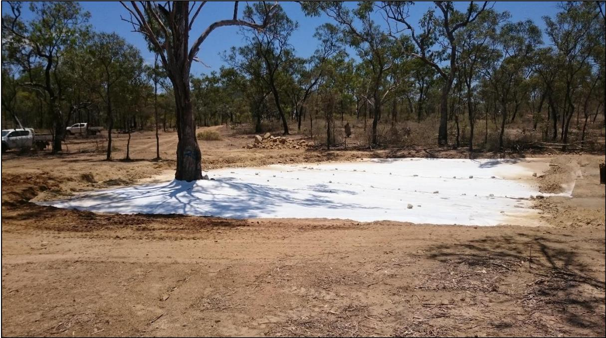
Figure S1-E. Geotextile fabric laid over former gully head scarp
