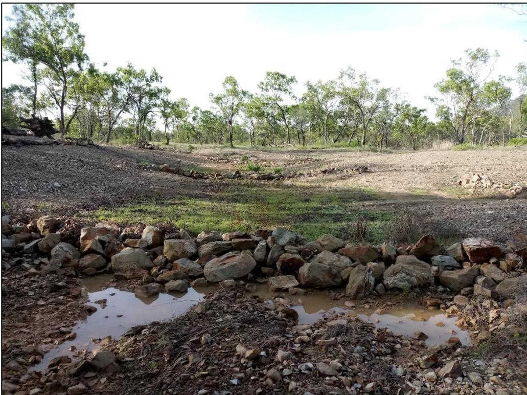
Figure SI-9C. Looking upstream into remediated gully at same location as Figure SI-9B. Photo taken in on 16/02/2018. Note the check dam has collected coarse sediment and now supports vegetation.
