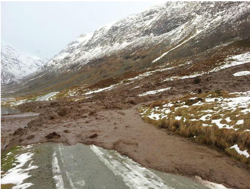
Figure S2: The debris flow deposits covered the road and continued into the lake. Photographed in the morning of 16 November 2013 by Vidar Leirdal.
