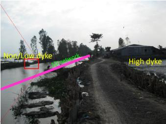
Figure 3. A high dyke and non/low dyke in An Giang province and their schematization in modelling. Photos by Vo Quoc Thanh 2012.
