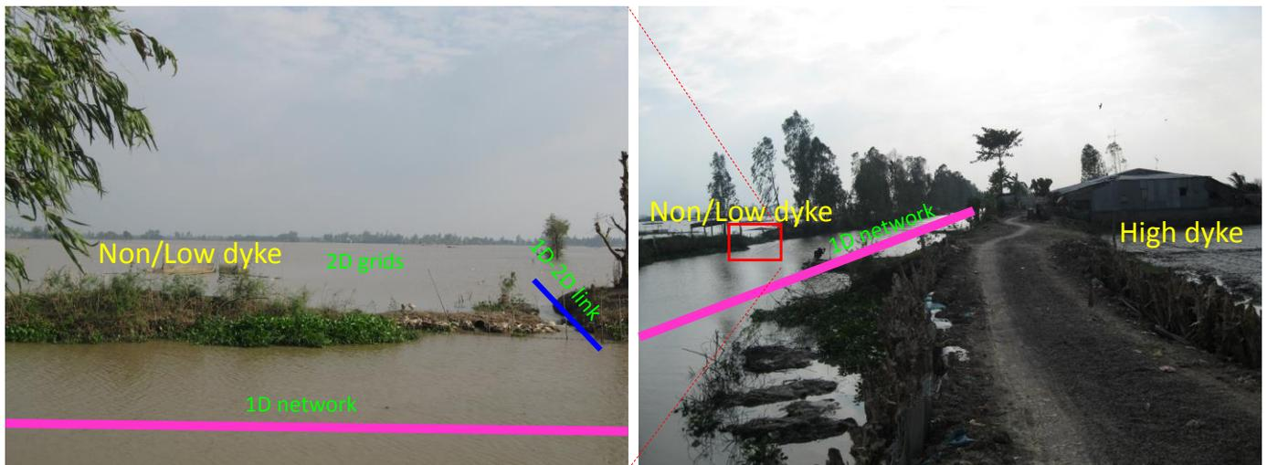
Figure 5. A high dyke and non/low dyke in An Giang province and their schematization in modelling. Photos by Vo Quoc Thanh 2012.
