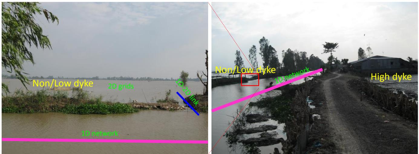
Figure 3. A high dyke and non/low dyke in An Giang province and their schematization in modelling. Photos by Vo Quoc Thanh 2012.
