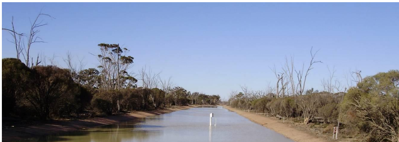
275 Figure 2: New broad-based channel implemented in Dulbinning Nature Reserve. Channel dimensions at this location are 23m wide, 0.55m deep. Water depth in this image is 0.18m.
