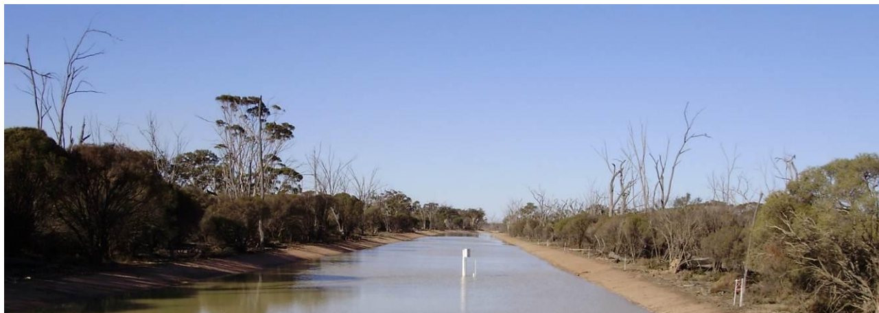
Figure 2: New broad-based channel implemented in Dulbinning Nature Reserve. Channel dimensions at this location are 23m wide, 0.55m deep. Water depth in this image is 0.18m.
