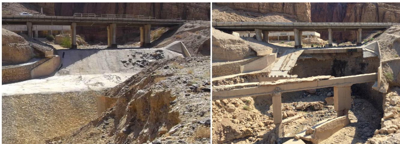
Figure 9: Example of a bridge along the Dead Sea motorway damaged by progressive erosion of the sediments. Similarly to Figure 8 A-B, all bridges along the coast are affected by the rapid incision of the river bed. Each year, the available energy released during erosion process is more important (square function)
