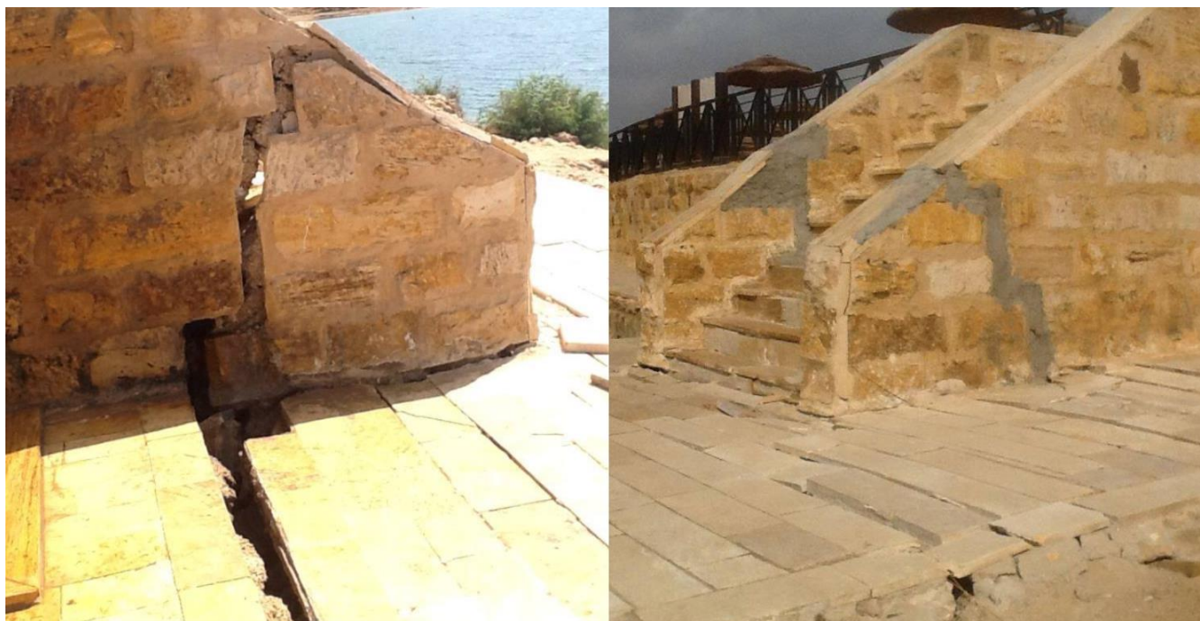
Figure 7: examples of damage (left) and o quick repair (right) in the front beach of the Movenpick hotel (south of Marriot Hotel).
