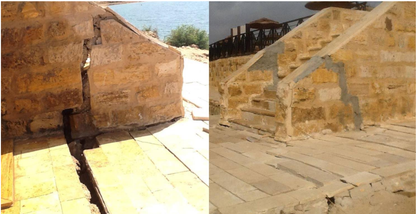
Figure 8. Examples of damage (left) and of quick repair (right) that are common in the beachfront of the hotels along the DS coastline.
