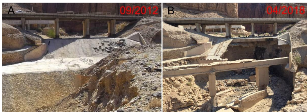
Figure 10. Example of a bridge along the Dead Sea motorway damaged by progressive erosion of the sediments. All bridges along the Dead Sea coast are affected by the rapid incision of the river bed.
