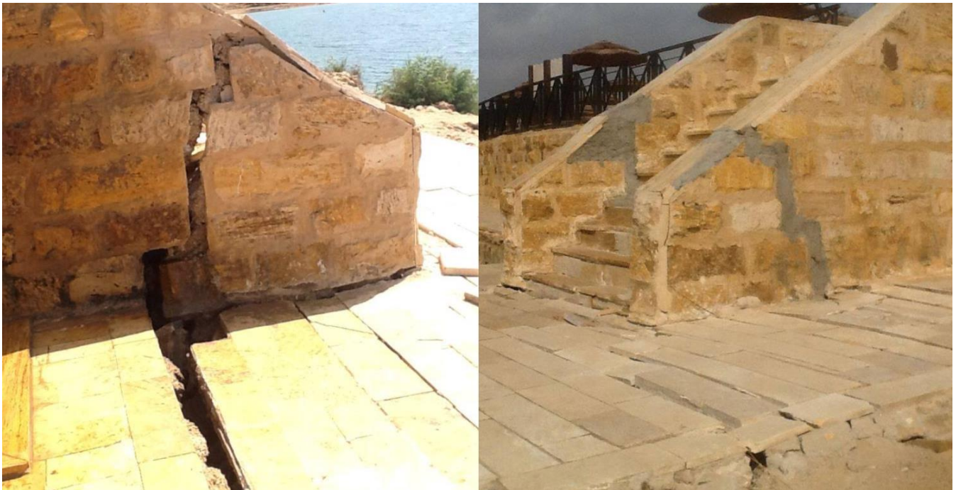
Figure 8. Examples of damage (left) and of quick repair (right) that are common in the front beaches of the hotels along the DS coastline.
