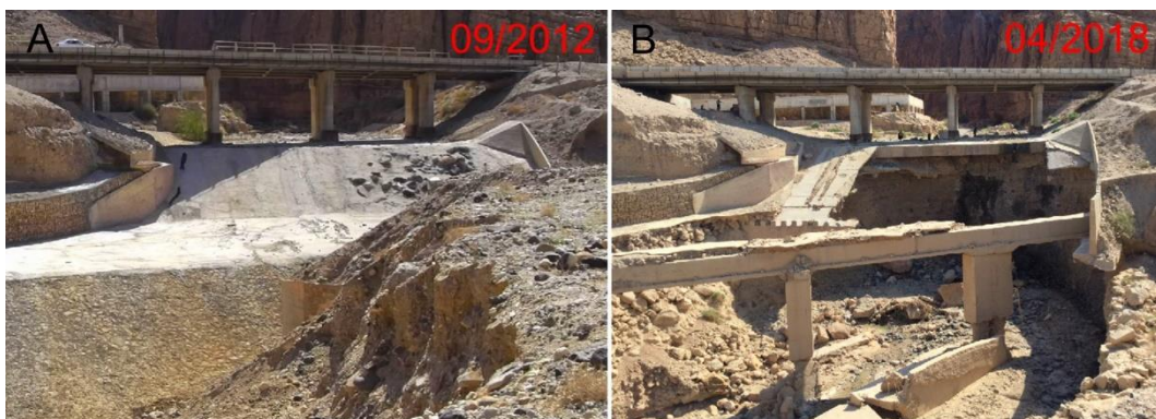
Figure 10. Example of a bridge along the Dead Sea motorway damaged by progressive erosion of the sediments. All bridges along the DS coast are affected by the rapid incision of the river bed. Each year, the available energy released during erosion process is more important (square function).
