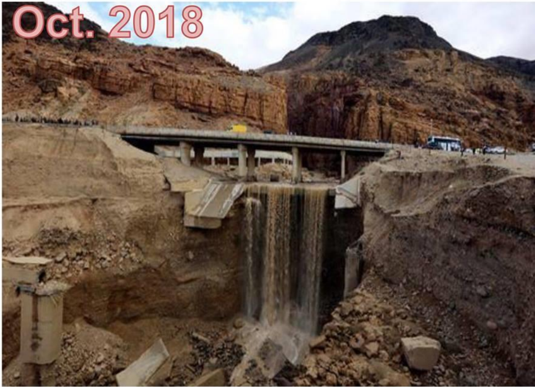
A partially damaged bridge which lost one of its pillars in Oct. 2017 leading to its partial closer. It totally collapsed on the 25th of Oct. 2018.
