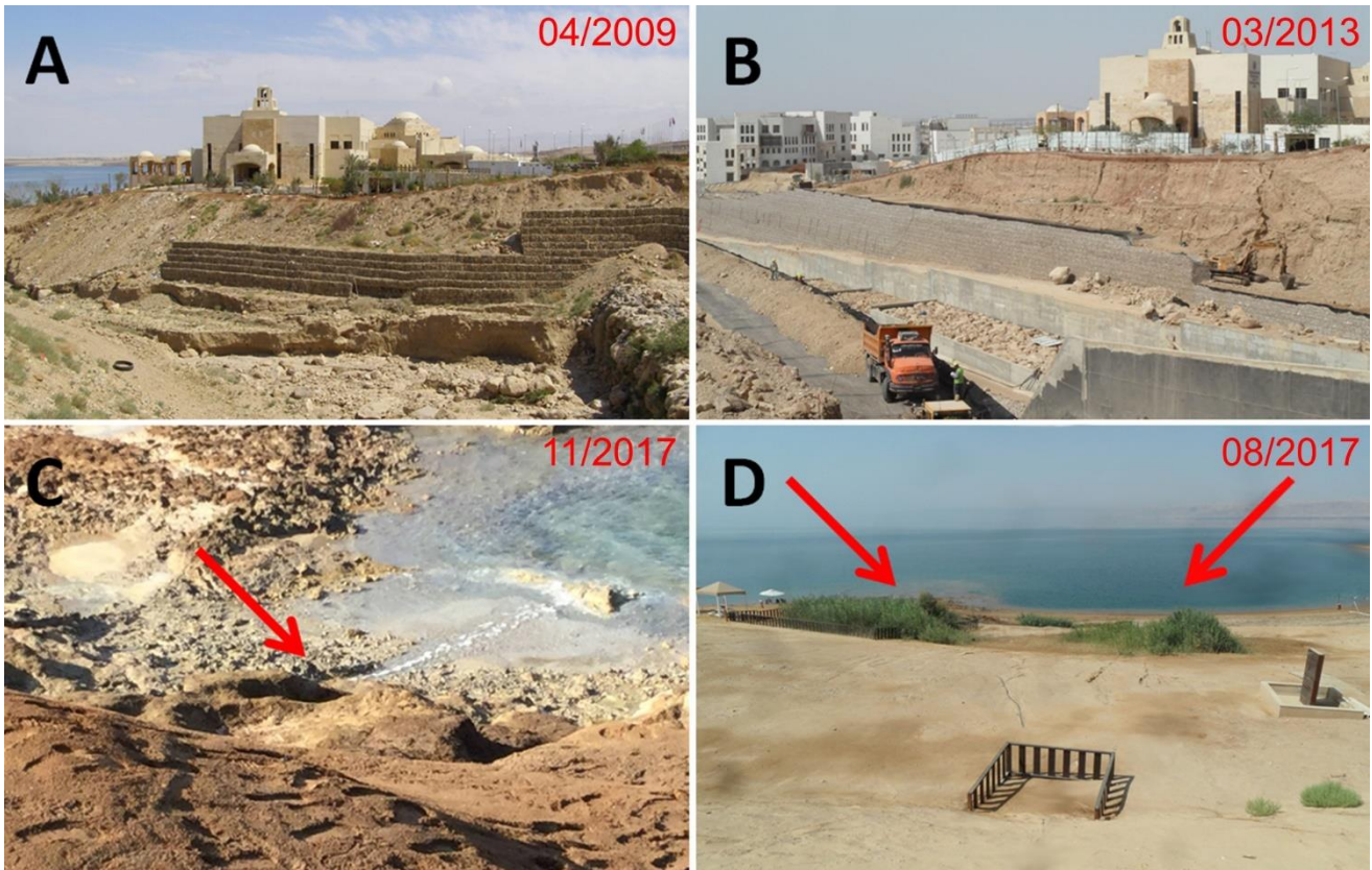
Figure 9. The King Hussein bin Talal convention centre and surrounding areas. a and b: the river next to the conference centre is entrenching at the same pace as the DS level lowering. Frequent works are needed to stabilize the slopes in the area. c: groundwater flowing under the convention centre.
