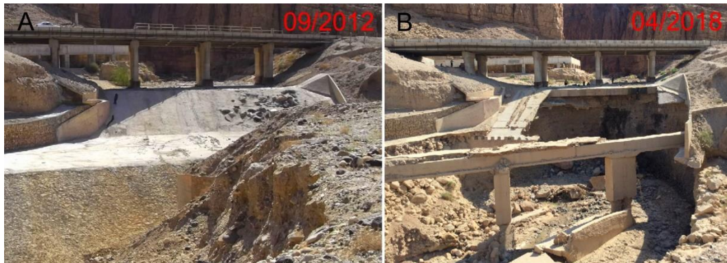
Figure 10. Example of a bridge along the Dead Sea motorway damaged by progressive erosion of the sediments. All bridges along the DS Dead Sea coast are affected by the rapid incision of the river bed. Each year, the available energy released during erosion process is more important (square function).
