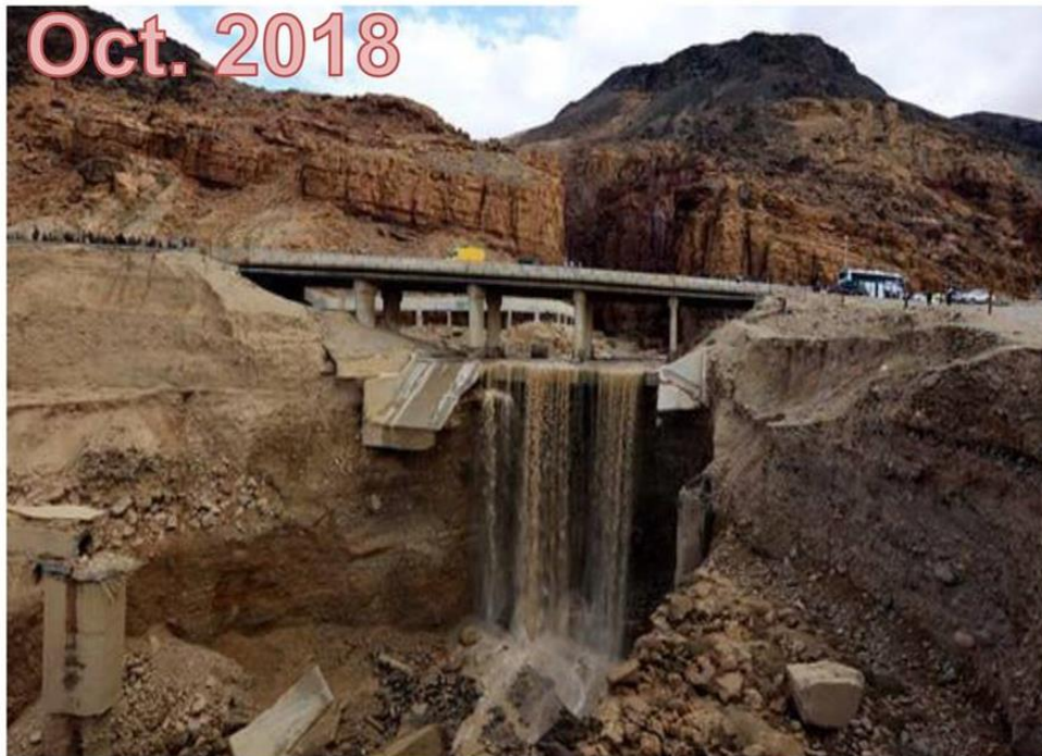
Figure 9: Example of a bridge along the Dead Sea motorway damaged by progressive erosion of the sediments. Similarly to Figure 8 A-B, all bridges along the coast are affected by the rapid incision of the river bed. Each year, the available energy released during erosion process is more important (square function)
