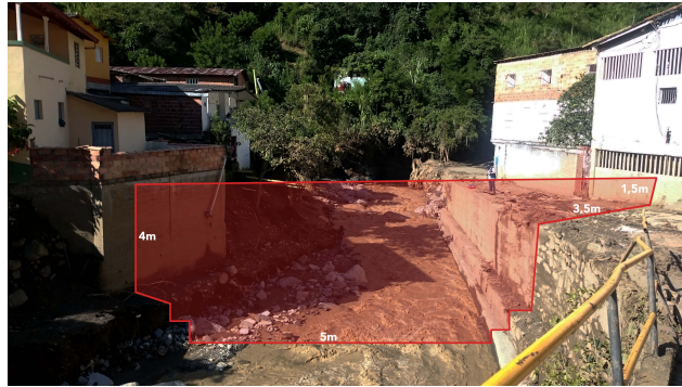
Figure 4. Channel cross-section showing an example of flooded infrastructure during the flash flood event. The section shows mud marks on the walls of adjacent houses, with heights varying between 0.5 and 1.2 m. The houses in the picture are located 4-5 m away from the channel. The photograph also shows the width of the channel and the total estimated depth during the flash flood. The cross-section is downstream from the bridge shown in the picture.
