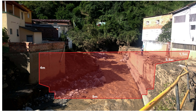
Figure 4. Channel cross-section shown an example of flooded infrastructure after the flash flood event. The section shows mud marks on the walls with heights varying between 0.5 and 1.2 m . These mud stains are evident in buildings located 4-5 m away from the channel. The photograph also shows the width of the channel and the total estimated depth during the flash flood.
