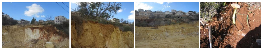
850 Figure A2. Soil cover – a, b & c) soil covering marly limestone with some white Nari crust (bottom Hebron/Top Yatta fn.); d) Ras Karkar terrace soil measurement site (lower Hebron fn.)
