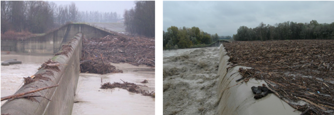
Fig. 3. Large wood debris accumulation on the Secchia flood control reservoir during a flood event close to the bottom openings (left) and on the overflow spillway (right).
