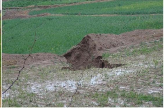
**Figure 3. Breached terrace bund/embankment**
