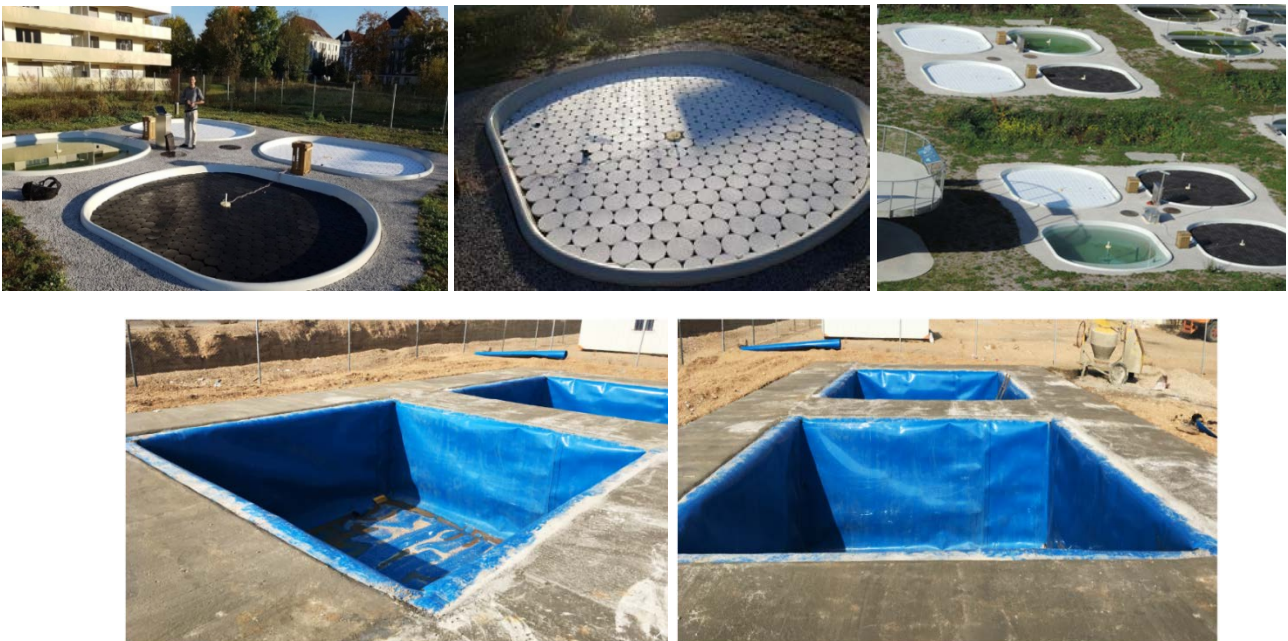
Figure D: Top: ongoing “field scale” experiments conducted in EAWAG near Zurich using 8 ponds each 14 \text{ m}^2 and 1.5 \text{ m} deep covered with white and black 0.2 \text{ m} (EVA foam) floating
