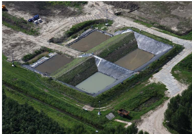
Figure 2: Large-scale piping facility
