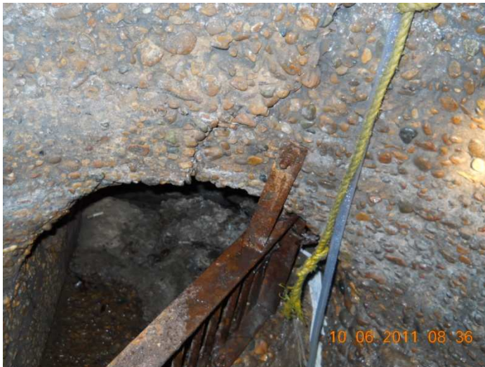
Fig 9: The bar screen is mounted securely over the dam.
