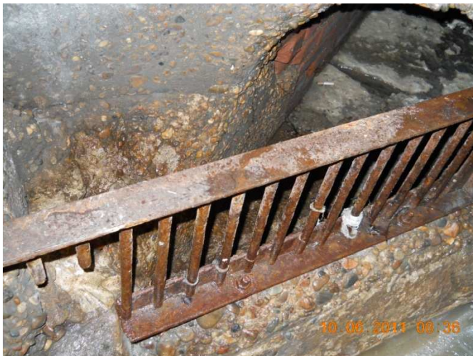
Fig 7: The bar screen is showing signs of rust but no major affects to its structural integrity.
