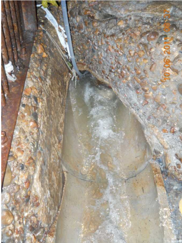
Fig 5: The downstream low flow line is in good condition
