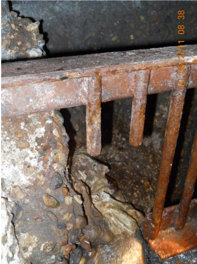
Fig 8: There is a space in the bar screen where debris could go through.
