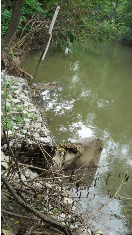
Fig 10: The tide flex valve is shut. There is no S & F near the site
