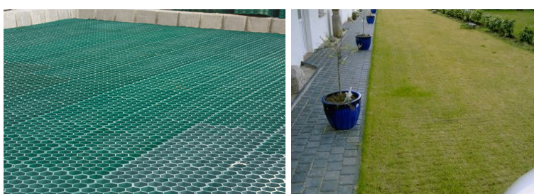
Figure S6: Pavement type D during installation (left) and inside the lawn (right).
