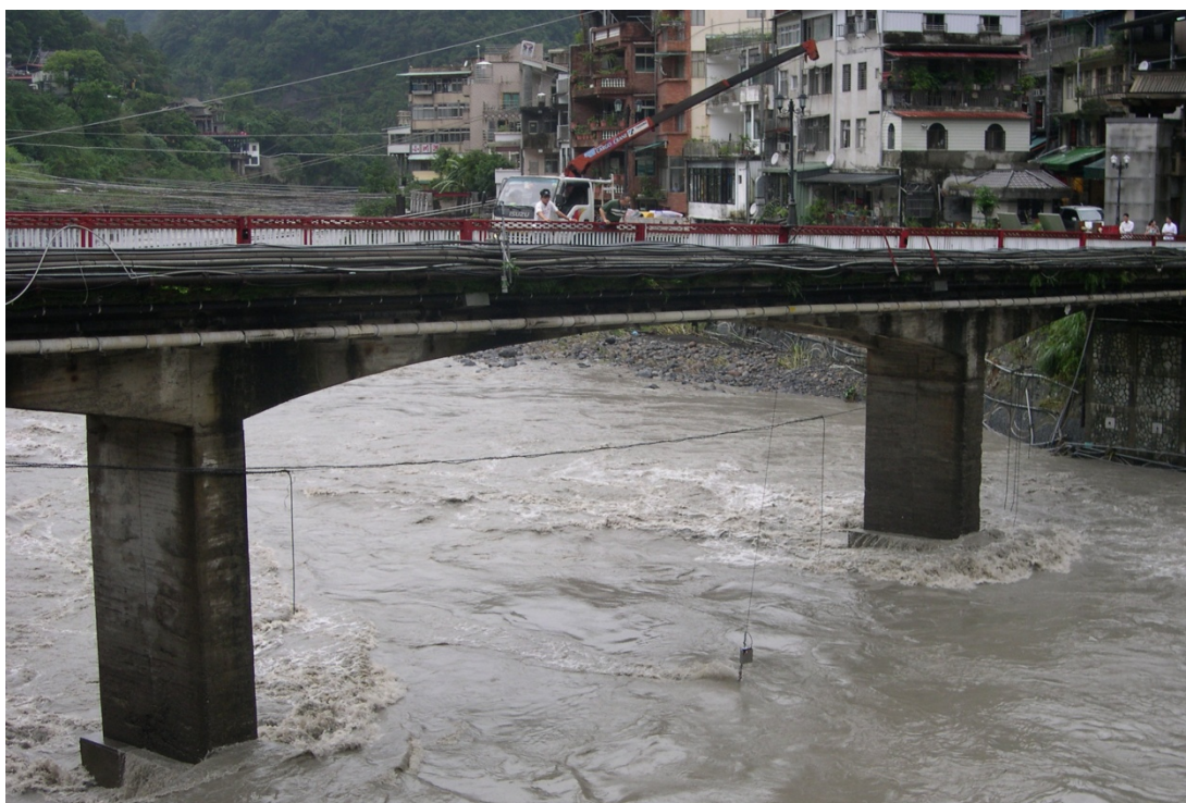
Fig. 3. Flood discharge measurement during Typhoon Krosa.
