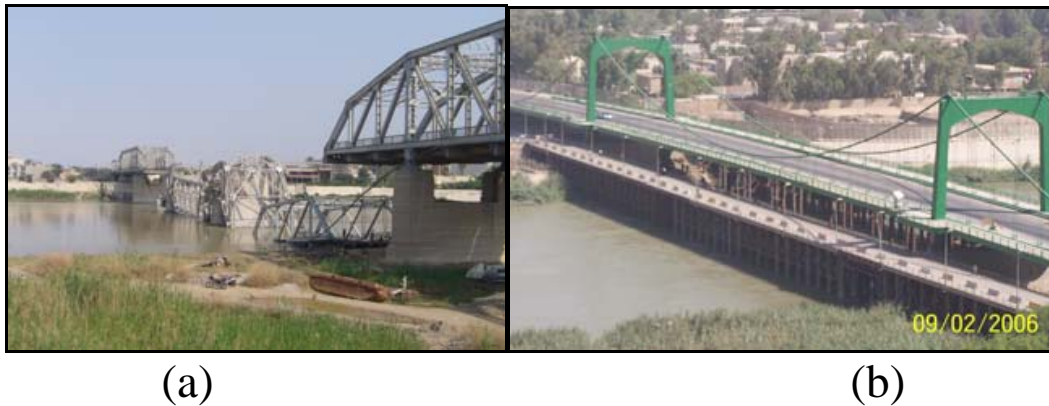
Fig. 3. (a) Destroyed parts from Al-Sarafiah Bridge have fallen in the river (from http://www.wikipedia.org ). (b) Temporary bridges parallel to the suspended bridge.
