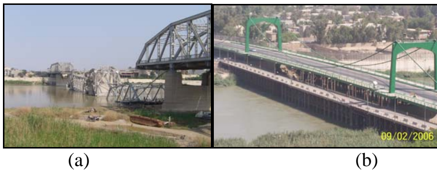
Fig. 3. (a) Destroyed parts from Al-Sarafia Bridge have fallen in the river (from http://www.wikipedia.org ). (b) Temporary bridges parallel to the suspended bridge.
