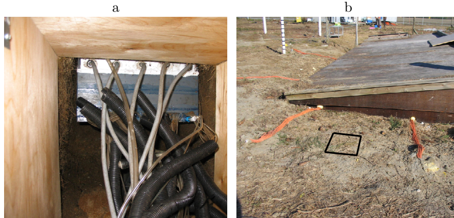
Fig. 1. Experimental setup. Installation of the multicompartment sampler (MCS), shown from the trench (a) . The location of the MCS shown from above (b) . The marked square indicates the location of the MCS, 51 cm below soil surface. The roof of the trench is visible in the background. The width of the MCS is 31.5 cm.
