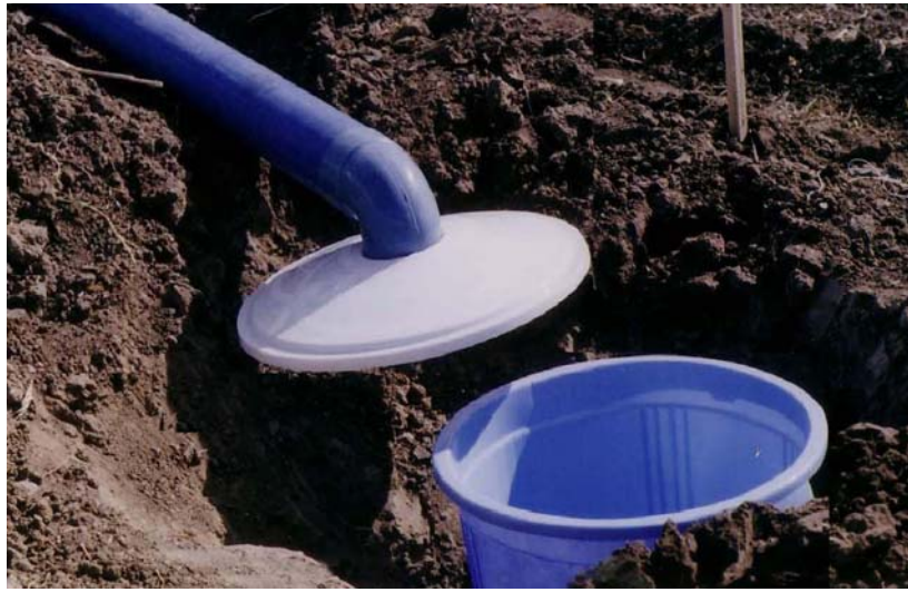
Fig. 3. Runoff-collecting installations consisted of gutter pipes, pipes and 70-l tanks at the lower part of the runoff plot
