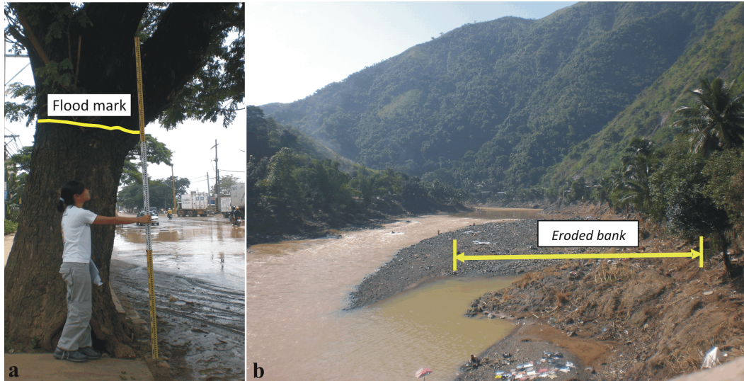
Fig. 3. (a) Photo taken along JP Rizal Avenue showing mud (stain) deposits on the bark of the tree indicating flood height and; (b) photo of upstream Marikina River showing extensive bank erosion.
