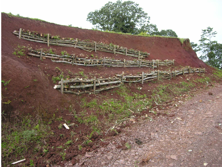
Fig. 9a. The live palisade just after construction.
