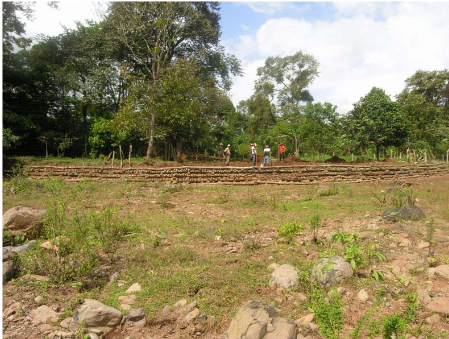
Fig. 9c. The vegetated crib wall along Wanawas river just after the construction.
