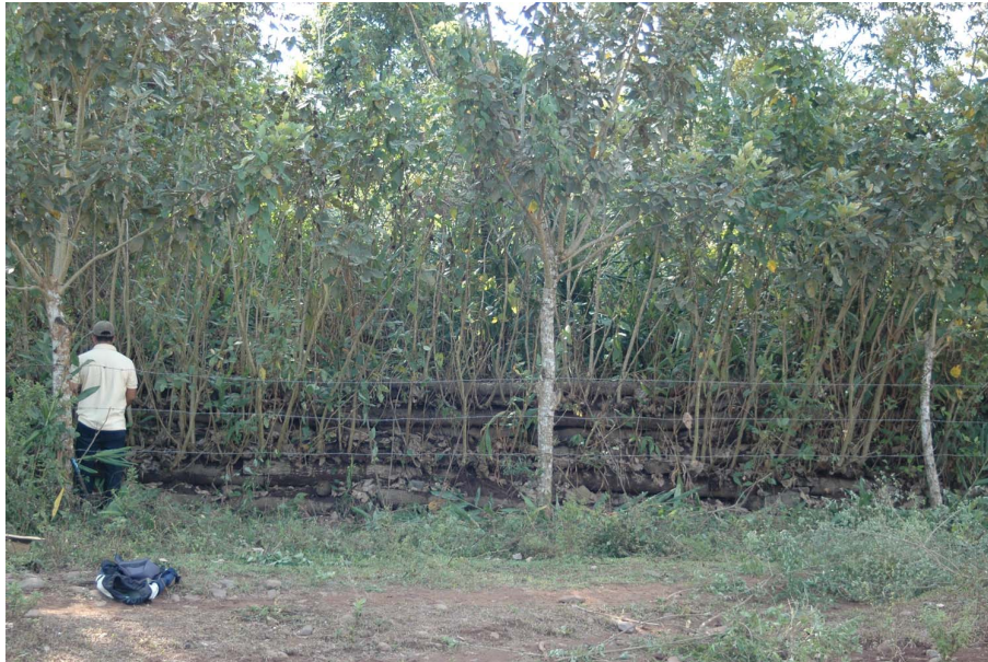
Fig. 9d. The vegetated crib wall one year after the construction.
