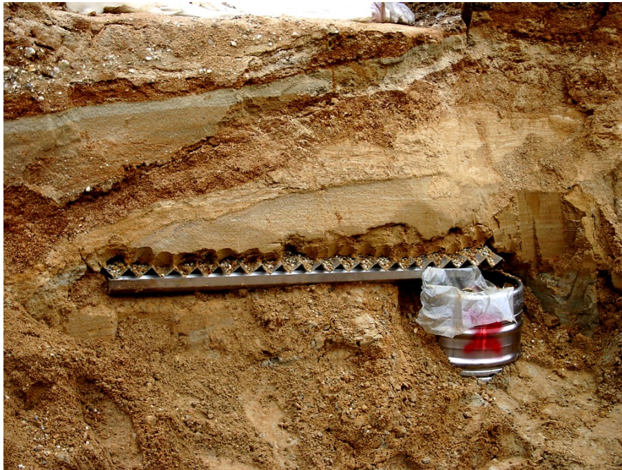
Fig. 2. Installed modular plate lysimeter prior to refilling of the access pit.
