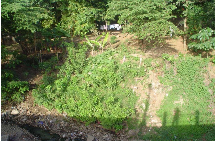
Fig. 8. The riverbank protection, 7 months after cuttings planted.
