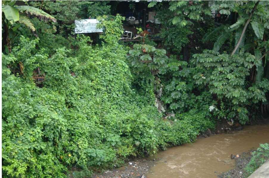
Fig. 10. The riverbank protection, 44 months after cuttings planted.
