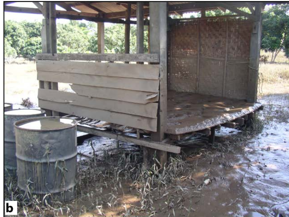
Fig. 8. (a) high water line on fruit trees. Floodwater depth was 1.3 m. Location is at point B of Fig. 11. View is to the southeast. (b) hut located at point H2 on Fig. 11. Five cm of sediment deposited on platform elevated 0.55 m above ground (see Fig. 12). Photos taken on 2 October.
