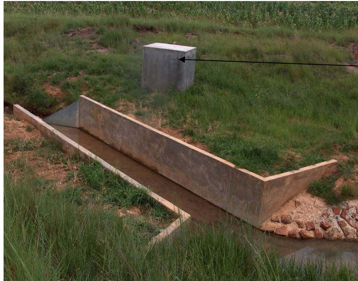
Fig. 4. An operational H-Flume in the Potshini catchment.
