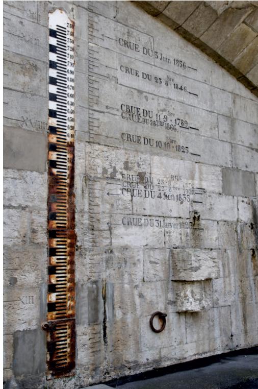
Figure 3. Historical flood marks of the River Loire in the Wilson Bridge in Tours (France). The elevations of the flood marks after the Direction regionale de l'environnement de l'Aménagement et du logement (DREAL), Centre-Val de Loire ( http://www.centre.developpement-durable.gouv.fr ). Discharge values associated to the flood levels after Duband (1996).
