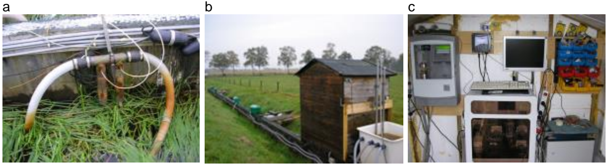
1 2 Figure 3: Pictures of the controlled drainage period setup, (a) the drainage overflow levels were 3 adjusted by attaching the flexible connection tube (with a SorbiCell socket between the black 4 fasteners) at the desired level, (b) the tube drain effluent was pumped to a collection vessel to 5 enable continuous monitoring of NO 3 -N and total-P concentrations using a Nitratax-sensor and a 6 Phosphax autoanalyser (c). 7
