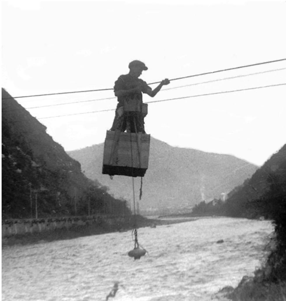
Figure 2: Stream flow measurements at the gauge station "Borgo a Mozzano" ( $43^{\circ} 59'30.73''\text{N}$ ;  $10^{\circ} 33'10.04''\text{E}$ ) in the River Serchio (Italy), probably taken in the 1920s or 1930s. The observer is placed in a box suspended on cable that moved along the cross section from which manages an old device to measure the stream flow velocity (Photo courtesy of Regione Toscana - Genio Civile di Bacino Toscana Nord e Servizio Idrologico Regionale).
