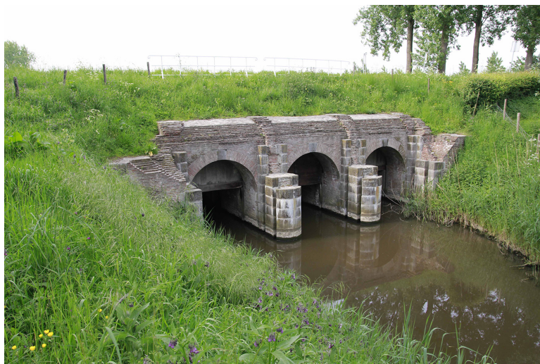
Figure 5. Land side of an inundation sluice, built in 1789 by the Estates General of the Dutch Republic at Zwartenhoek (51°15' N and 3°51' E). Notice the double groove in the protruding parts in which beams could be installed. As the space in between the beams could be filled with earth, this construction was strong enough to prevent the fresh water from flowing seaward. After some weeks water in polders could reach a level of some decimeters. As soon as the threat of war disappeared, beams and earth were removed again (photo, Nellie de Kraker).
