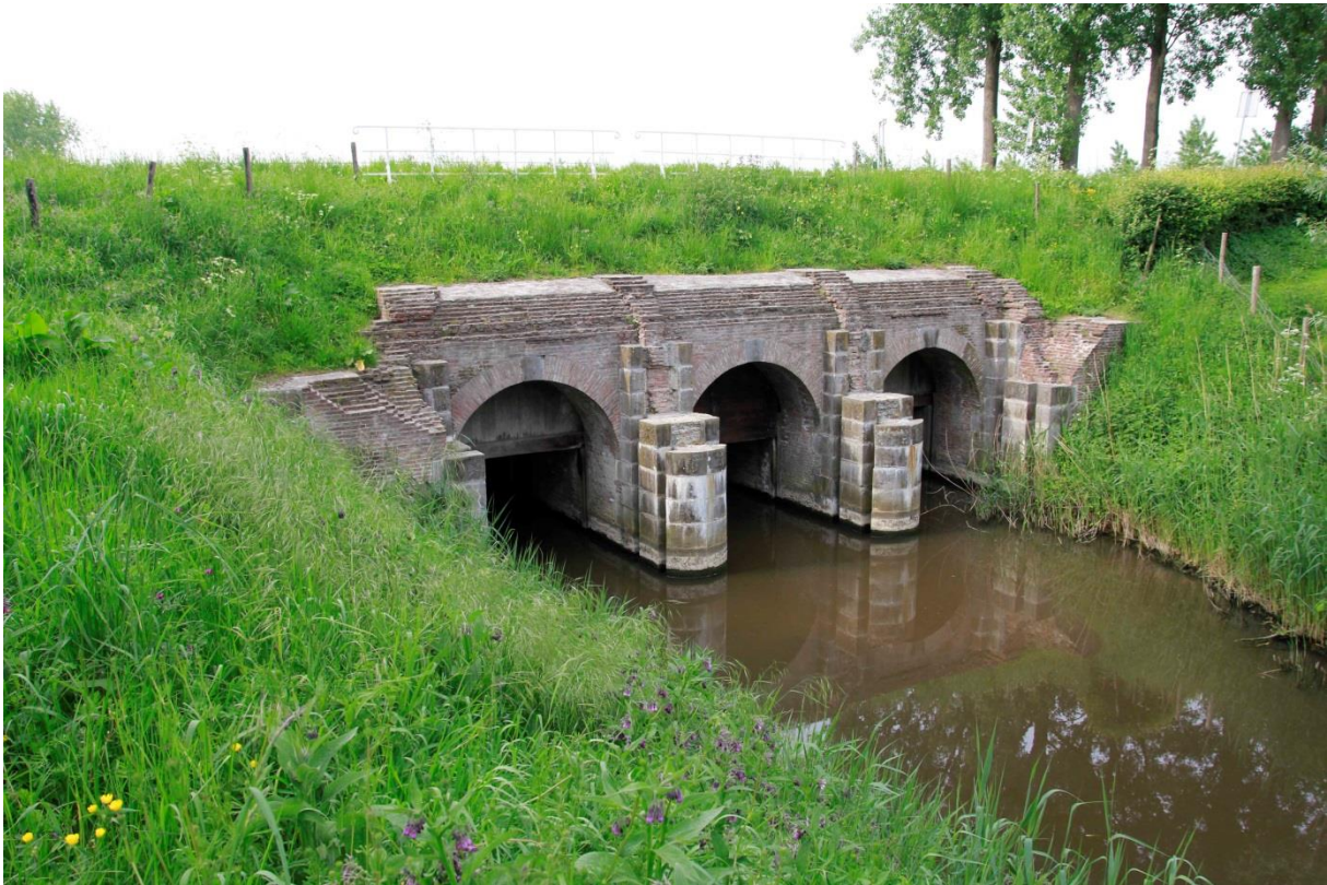
659 Fig. 5. Land side of an inundation sluice, built in 1789 by the Estates General of the Dutch Republic at 660 Zwartenhoek (51°15' N and 3°51' E). Notice the double groove in the protruding parts in which beams 661 could be installed. As the space in between the beams could be filled with earth, this construction was 662 strong enough to prevent the fresh water from flowing seaward. After some weeks water in polders 663 could reach a level of some decimeters. As soon as the threat of war disappeared, beams and earth 664 were removed again (photo, Nellie de Kraker).
