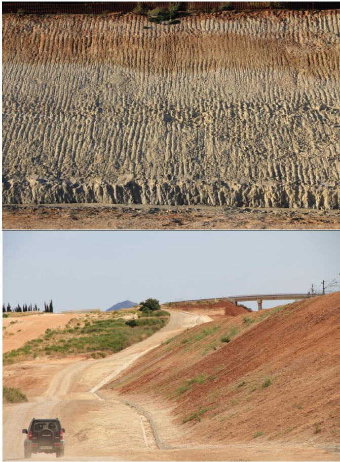
Figure 4. Photographs of the road and railway embankments studied. Note the lack of vegetation cover in both photographs and prominent rill development in the upper photograph.
