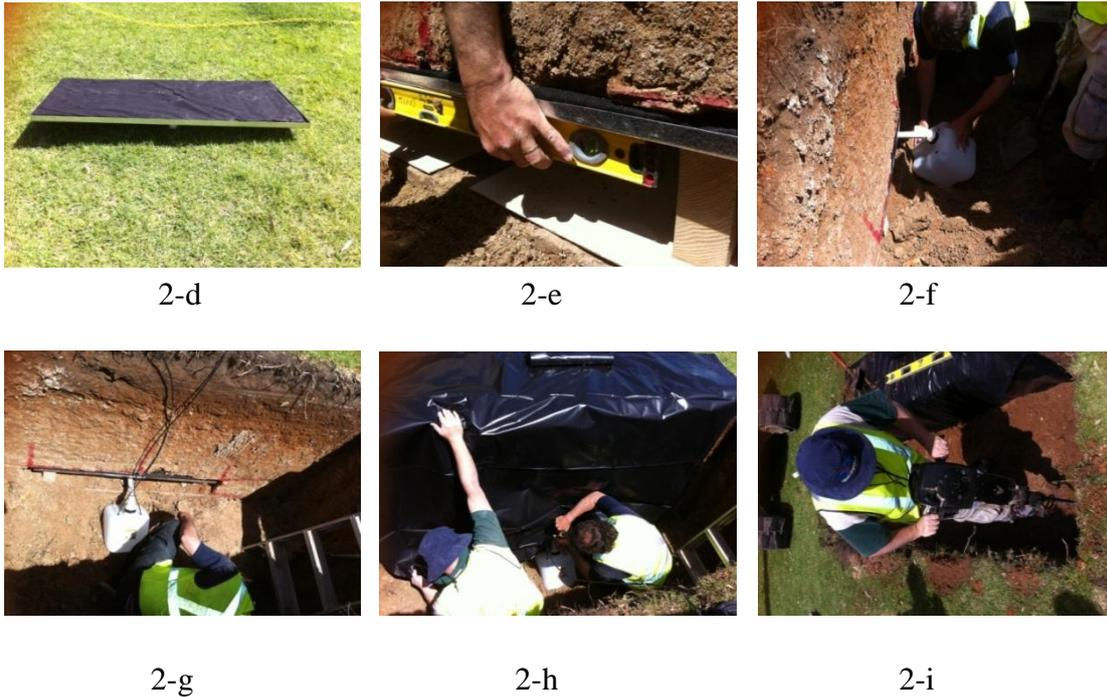
Fig. 2 Pan lysimeter installation, 2-a trench excavation, 2-b cavity digging, 2-c cavity levelling, 2-d lysimeter tray, 2-e placing the tray, 2-f placing the collecting bucket and connect the tray and bucket by a PVC pipe, 2-g PVC pipe and access tubes, 2-h plastic sheet for protecting the cavity, 2-i compacting the backfilled soil.
