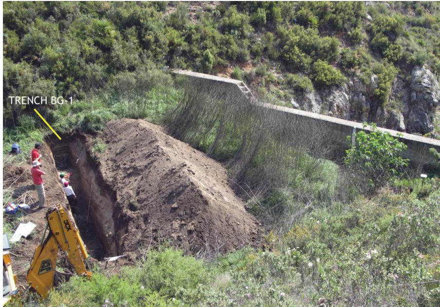
Fig. 5. The reservoir trench BG-1, closest to the dam.
